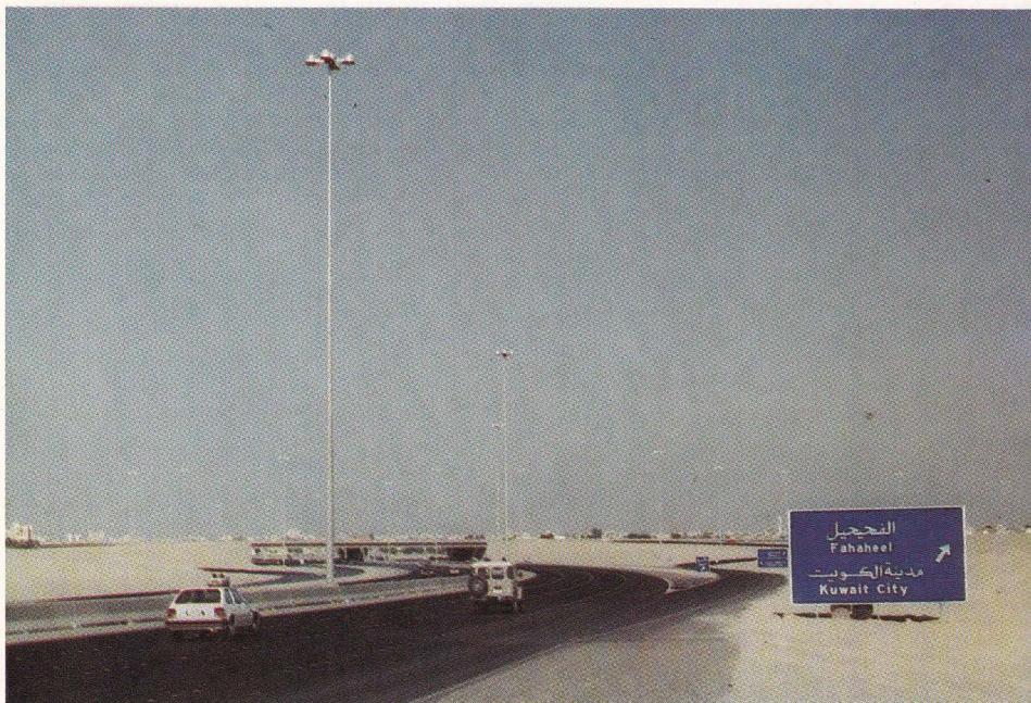
Kuwait Motorway. 30 metre Masts with 1000W MBI lanterns.
