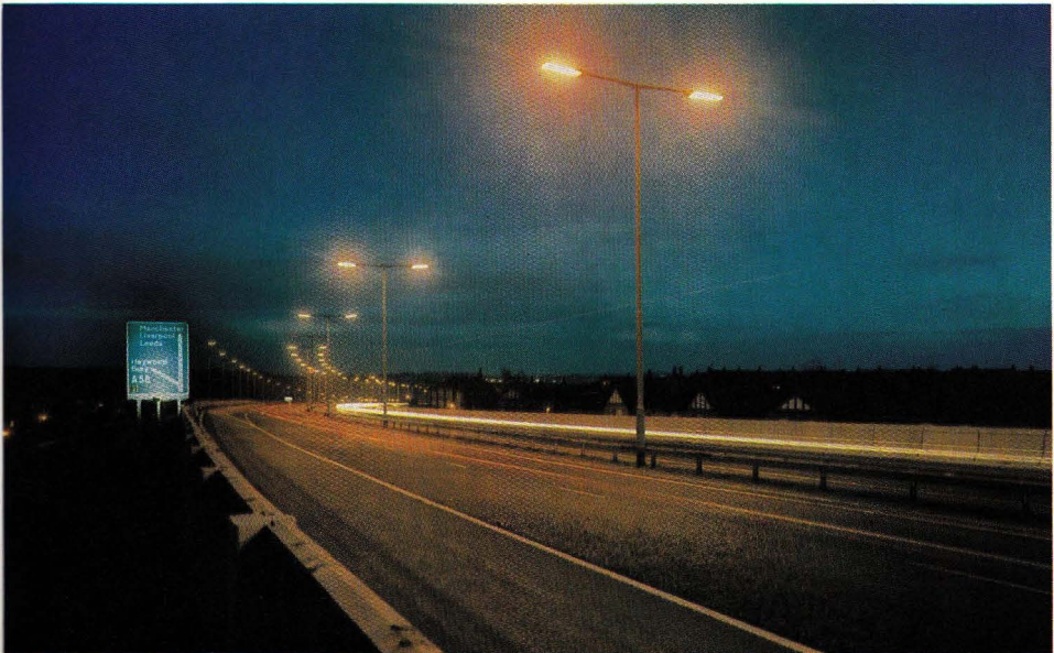
M62 Motorway, Manchester, using 180W Super SOX lamps and Z9563 lanterns.
