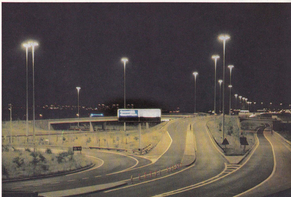
Renfrew Motorway, Glasgow. 18 to 36 metre Masts with 400W Solarcolour lanterns.
