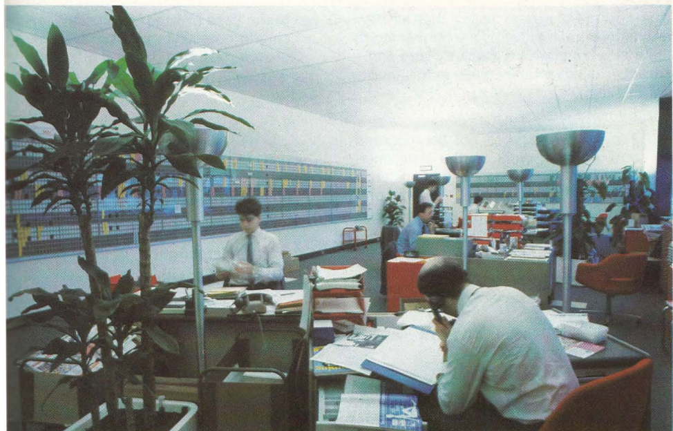
Uplighters with 250W Solarcolour De Luxe lamps provide efficient, glare-free lighting for colour printers Hunterprint at their Corby based offices.
