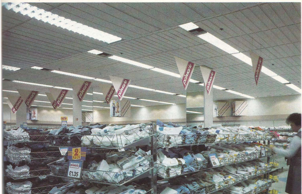
The Brighton Primark store features continuous lines of recessed fluorescent fittings which include air handling facilities and low brightness louvres.
