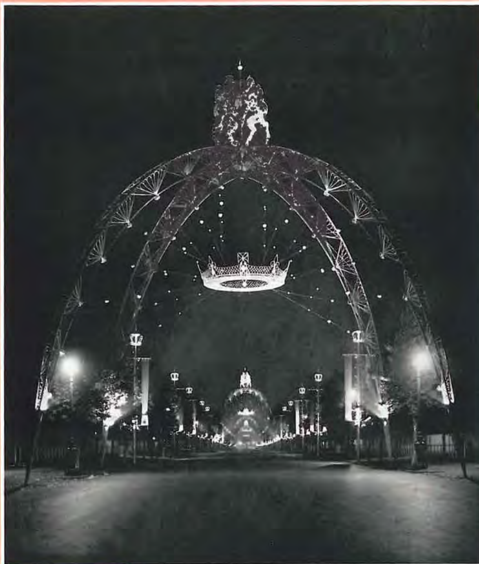
The Triumphal Arches in The Mall with Ministry of Works decorative lighting in which Philips 'Altrilux' high intensity internal reflector lamps were used to light the Arches and the Coronet from within the legs of the Arches themselves.
