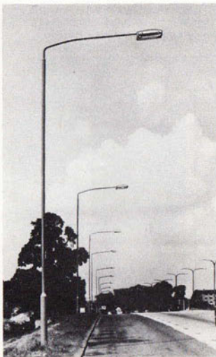
QA10.D.1090 on 8 metre steel column
