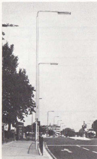
QA5.1200 on QLC.M0887 steel column
