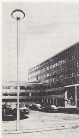
QG4.0/W3400 on a QLCH.0860/G4/DB Steel Column.
